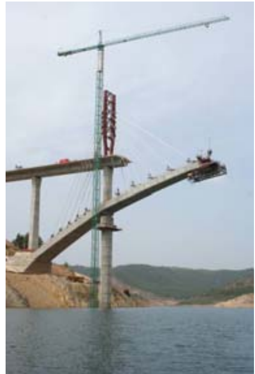
Fig 6. Pila provisional
